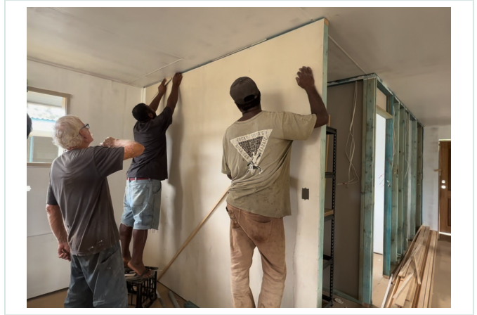
Local builders completing the clinic interior.
