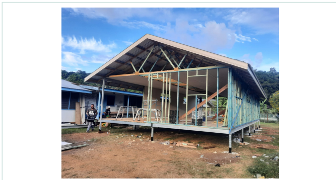
The prefabricated frame taking shape beside Kirakira Hospital.
