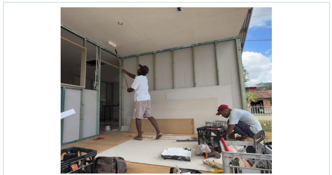
Local builders installing the external cladding.
