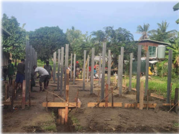
The construction at the end of the first week.
